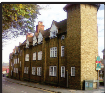
GUILDFORD 26 apartments Full service charge management
